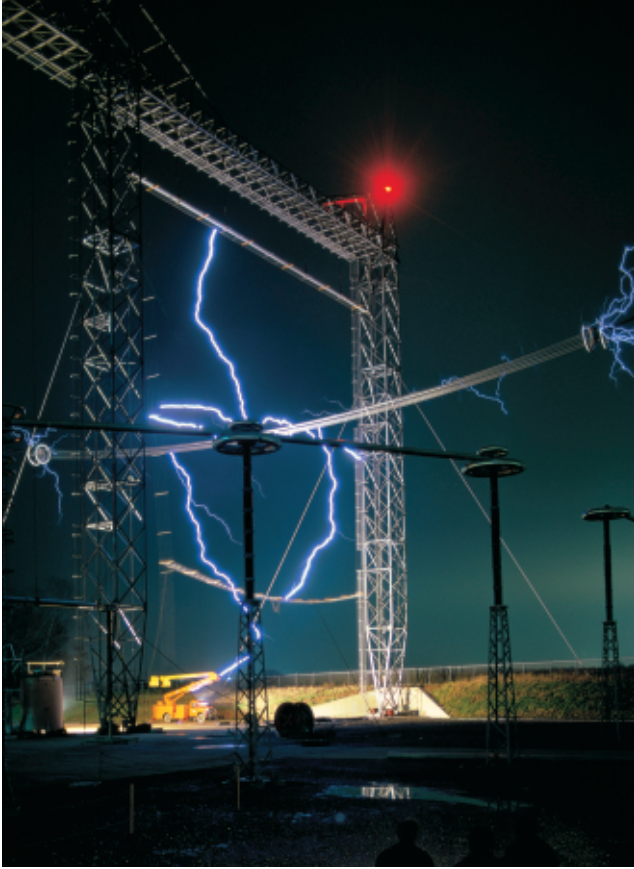
Figure 5 An outdoor ultra-high-voltage laboratory generates artificial lightning to test its effects on electrical utility equipment.
